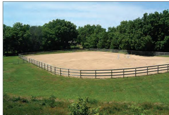
**Figure 5-2** Outdoor arena with good drainage. This arena is located at a higher elevation than the surrounding area. The ground is sloped away from the arena, which helps in drainage.
