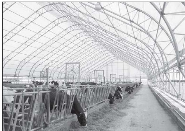
**Figure 16. Inside of a four-row freestall barn with an interior feed platform.**
