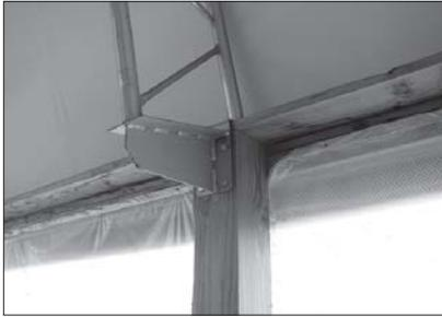
**Figure 18. Hoop frame connection to post frame wall.**
