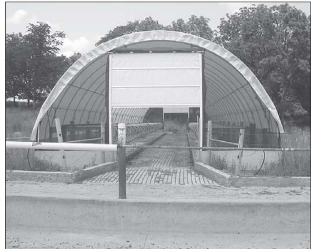
**Figure 9. Outside of a two-row hoop freestall barn.** Photo shows the feed platform side of the structure for the layout in Figure 8. Note wind shade cloth end wall ventilation and roll-up door for cow and equipment access.
