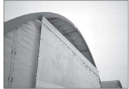
**Figure 24. Hoop frame connected to endwall.**
